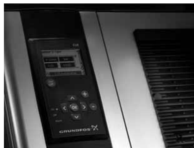
Fig. 22 Grundfos CUE control panel
